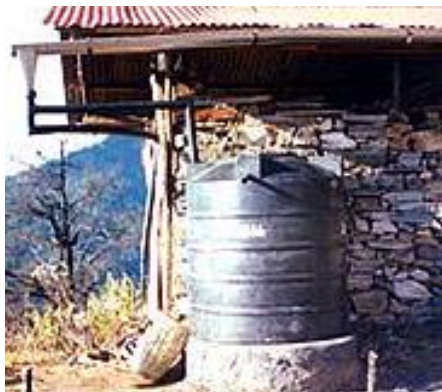
Figure VI-2 Rain Water Harvesting
